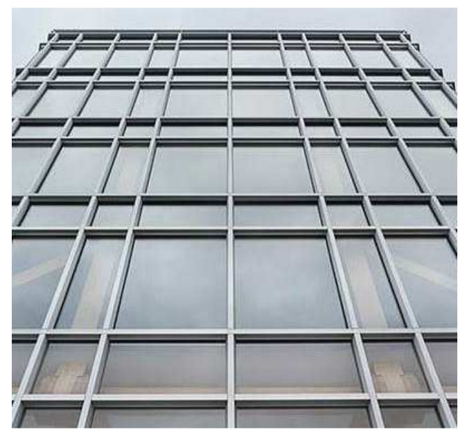
AF01 ALUMINIUM FRAME ON FACADE
